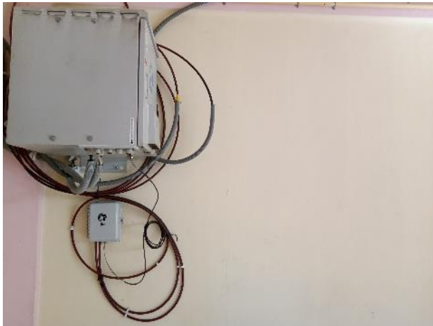
Reliance JIO access points located at various places in the campus for Wi-Fi
