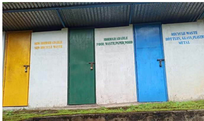
OVERVIEW OF WASTE SEGREGATION UNIT
